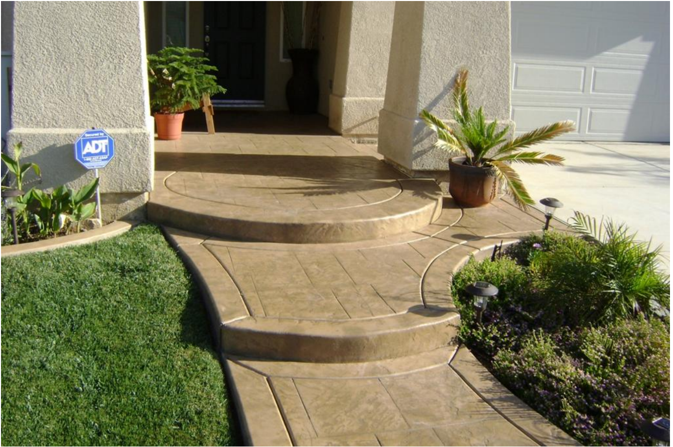
The photograph above is custom concrete path/steps that transform an entryway.
