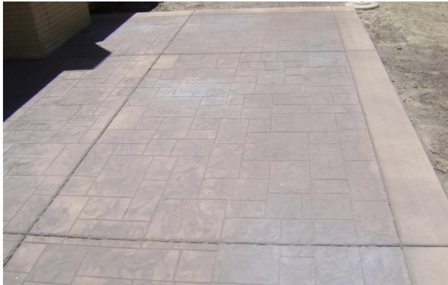
The photograph above is stamped concrete before it is sealed.
