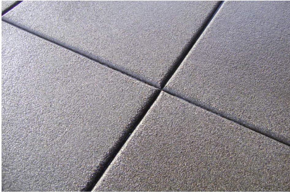
The photograph above is concrete path with an acid wash.
